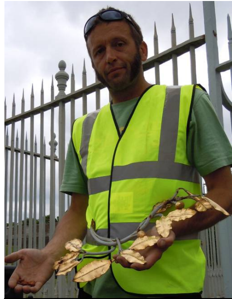
The fixings holding this leafwork overthrow were failing and were removed for safety and repair by Alex Coode.
