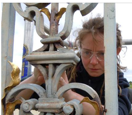
Jo Adkins removing paint to expose hidden corrosion.
